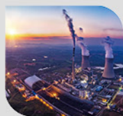
Environmentally friendly heating
