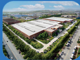
Laishan Industrial Park
