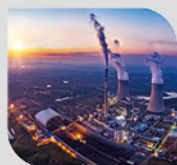
Environmentally friendly heating
