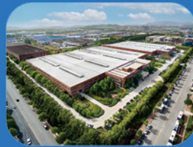
Laishan Industrial Park
