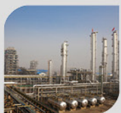
Energy and chemical equipment
