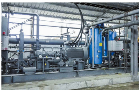
Synthetic ammonia low-temperature methanol washing CO 2 recovery and liquefaction project
