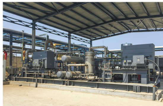
Water-cooled two-stage compressor unit
