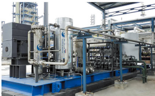
Engineering project of catalytic cracking flue gas recovery of 100,000 tons of liquid CO 2
