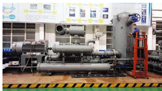
Ammonia compressor unit project for H 2 S purification unit
