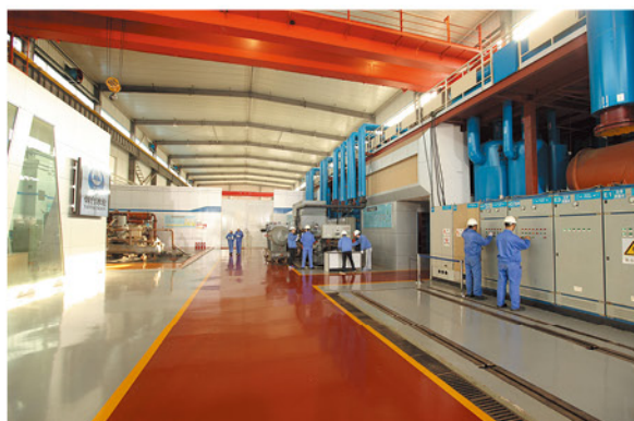
Comprehensive Performance Test Center
