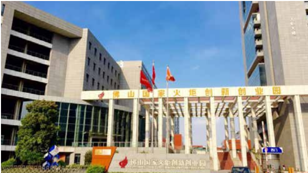
Foshan National Torch Innovation Park
