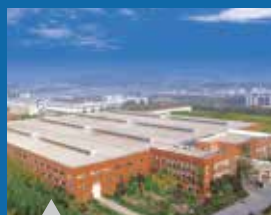
Laishan Industrial Park
